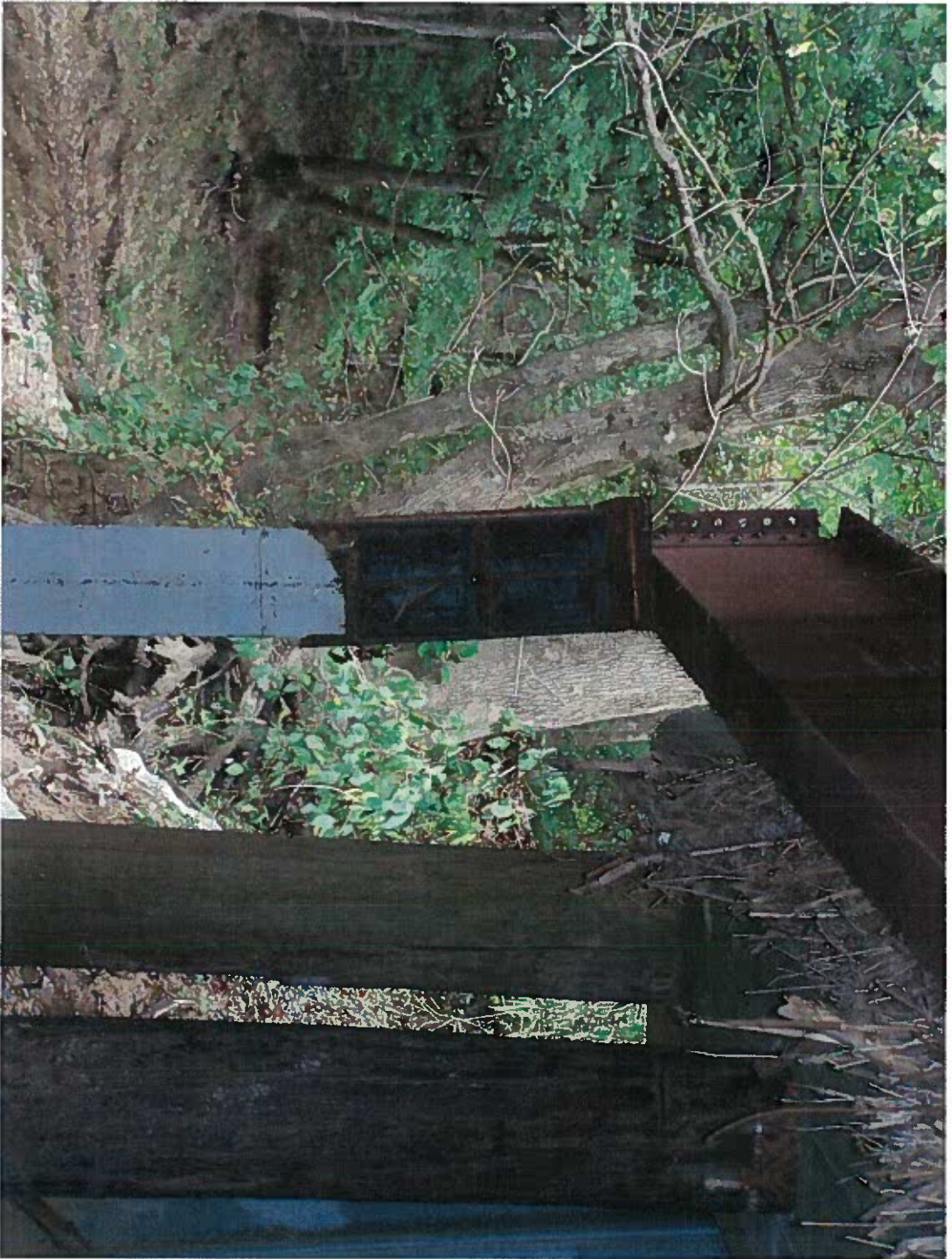
Bent 2, uspsream side false bent support
